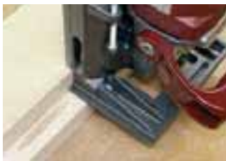
Repair in the groove
