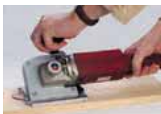
Planing protruding patch
