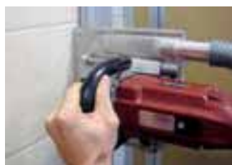
Cut into the tiled wall
