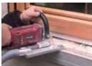
Cut-out for the weatherboard
