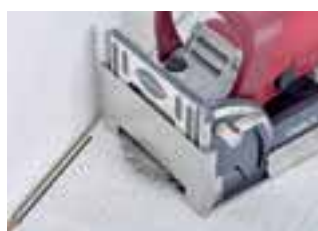
Cut expansion gaps
